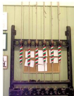
Ellacombe chiming apparatus with mini sallies at St Martin's
